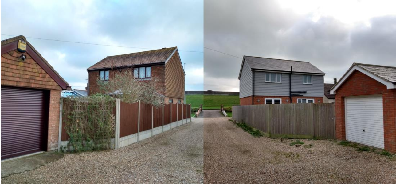
Photo 4: Rear of 1 and 2 Willop Close
