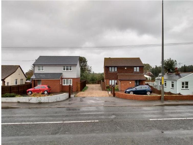
Photo 1: 1 and 2 Willop Close with site access between.
